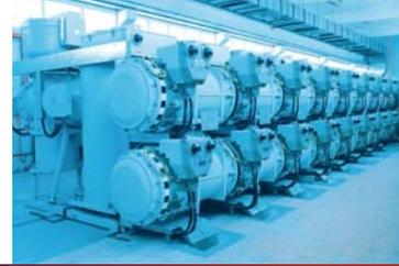
Rapid detection of SF<sub>6</sub> leaks with non-radioactive source helping to reduce emissions and protect the environment.
